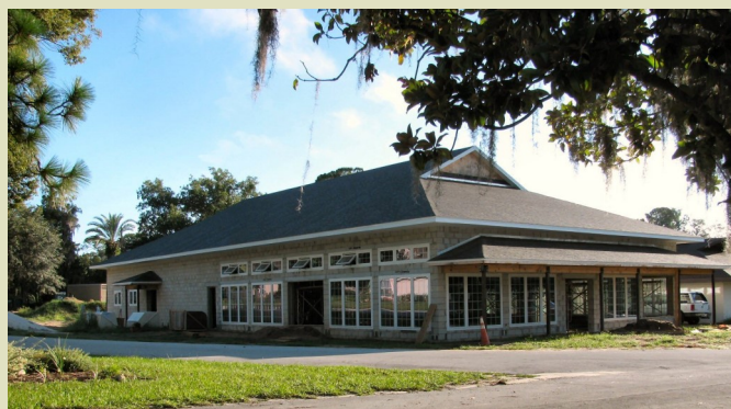
Progress continues on the Activity Building
