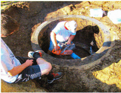
Installing a water pressure reducing valve
